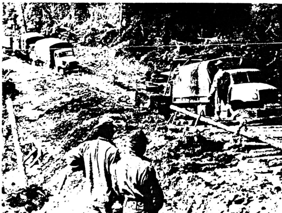
During the highway's construction, engineers removed muskeg and topsoil, then backfilled with gravel and rock, which promptly sank into the mud when the roadbed thawed. Swampy sections of the highway were turned to quicksand by rain. Hundreds of miles of road were corduroyed. (Courtesy of Yukon Archives)
